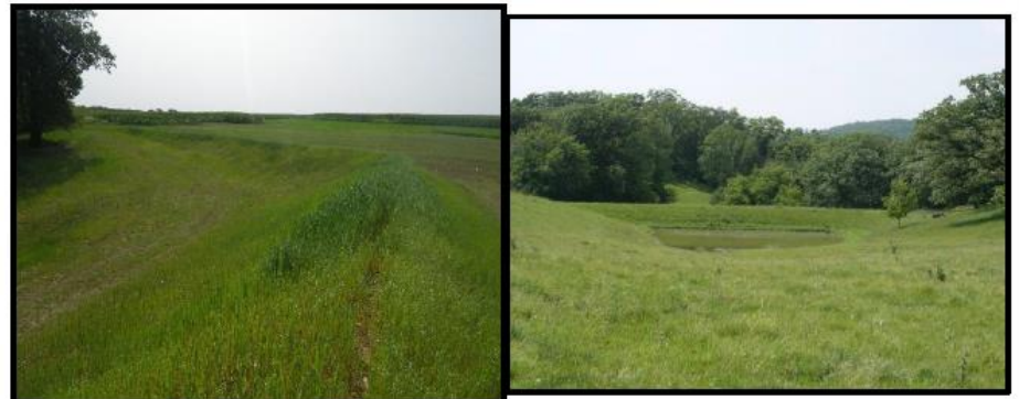
3 Implementing the BMPs (ex: Sediment Basin and Grade Stabilization Structure)
