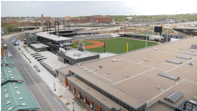
Rainwater is collected from the Metro Transit roof on the lower right for toilet flushing and irrigation at the stadium in the upper left.
