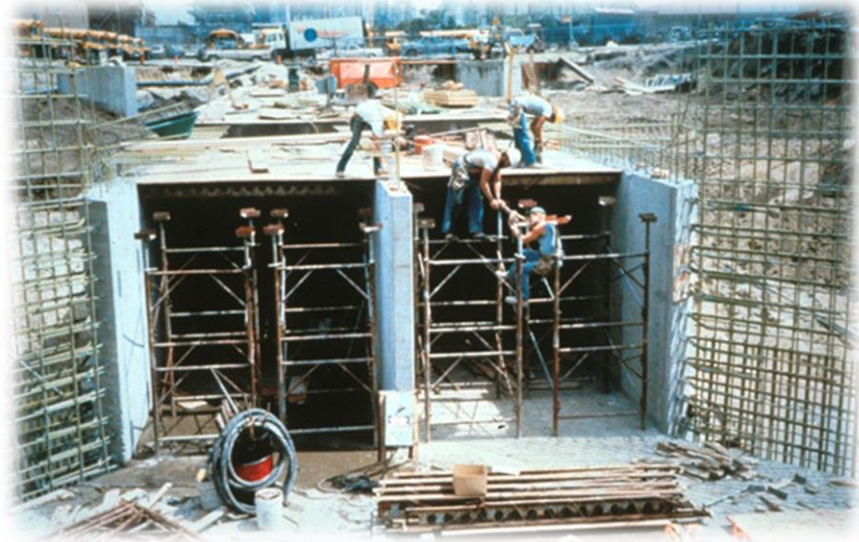
Double Box Culvert 1992
