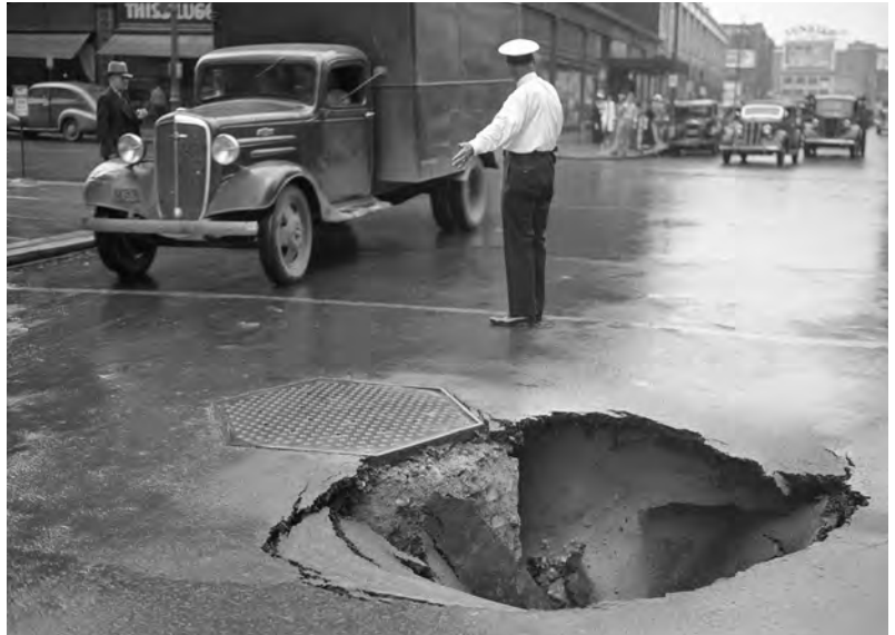
Sinkhole in a downtown Minneapolis street caused by a spring storm. Minneapolis Star and Tribune Company June 16, 1937, from the Minnesota Historical Society.
