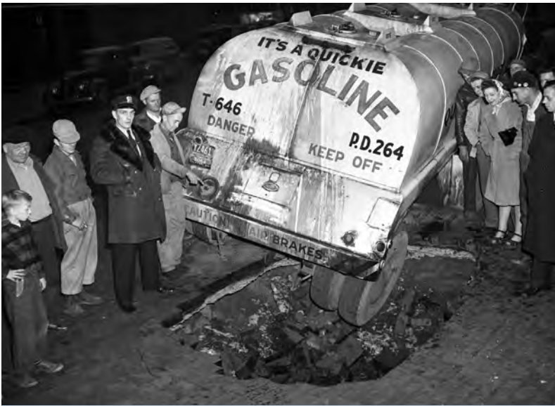
A gas tanker that hit a sinkhole in Minneapolis, 1946. Credit: Minnesota Historical Society.
